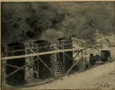
Each of the big tanks holds over 5,000 gallons but less than two gallons of oil are produced for each 5,000 gallons of water pumped into them.
